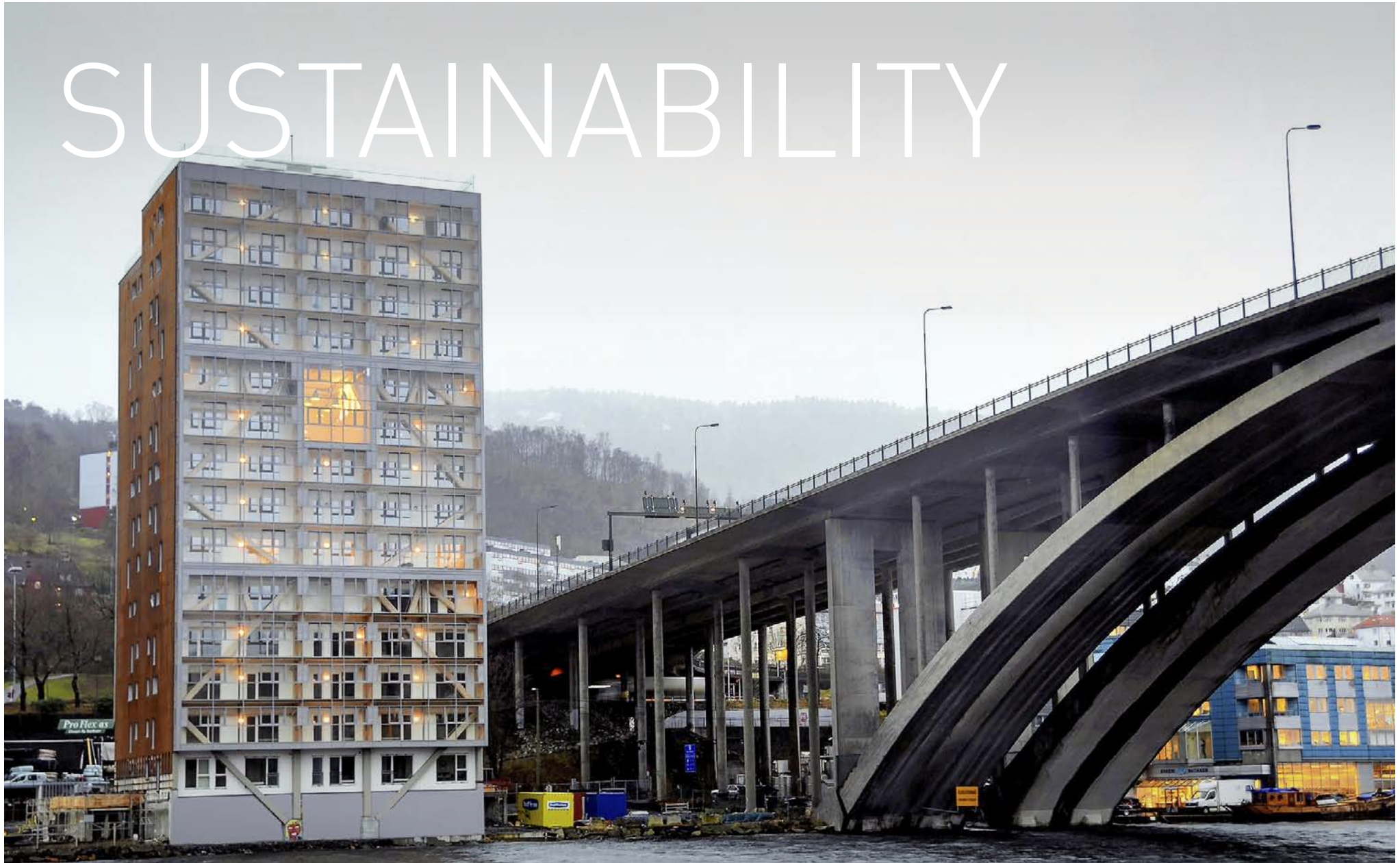
The world's tallest wooden house "Treet" in Bergen, Norway with ROCKWOOL facade insulation contributing to the apartments being built according to passive house requirements.
